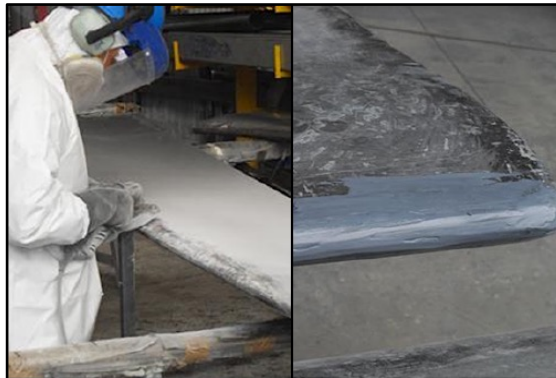
In process: blade in prep stages and partial ARC 858 repair.
